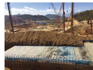
Dali East sea developing zone Utility tunnel
