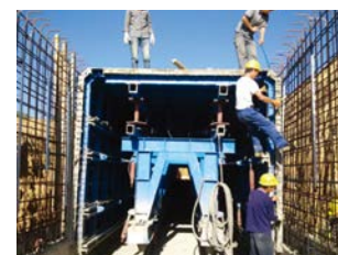
Dali East sea developing zone Utility tunnel
